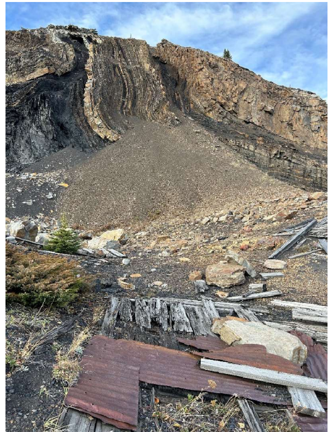
Previously mined open pit with former underground mine entry and associated debris
