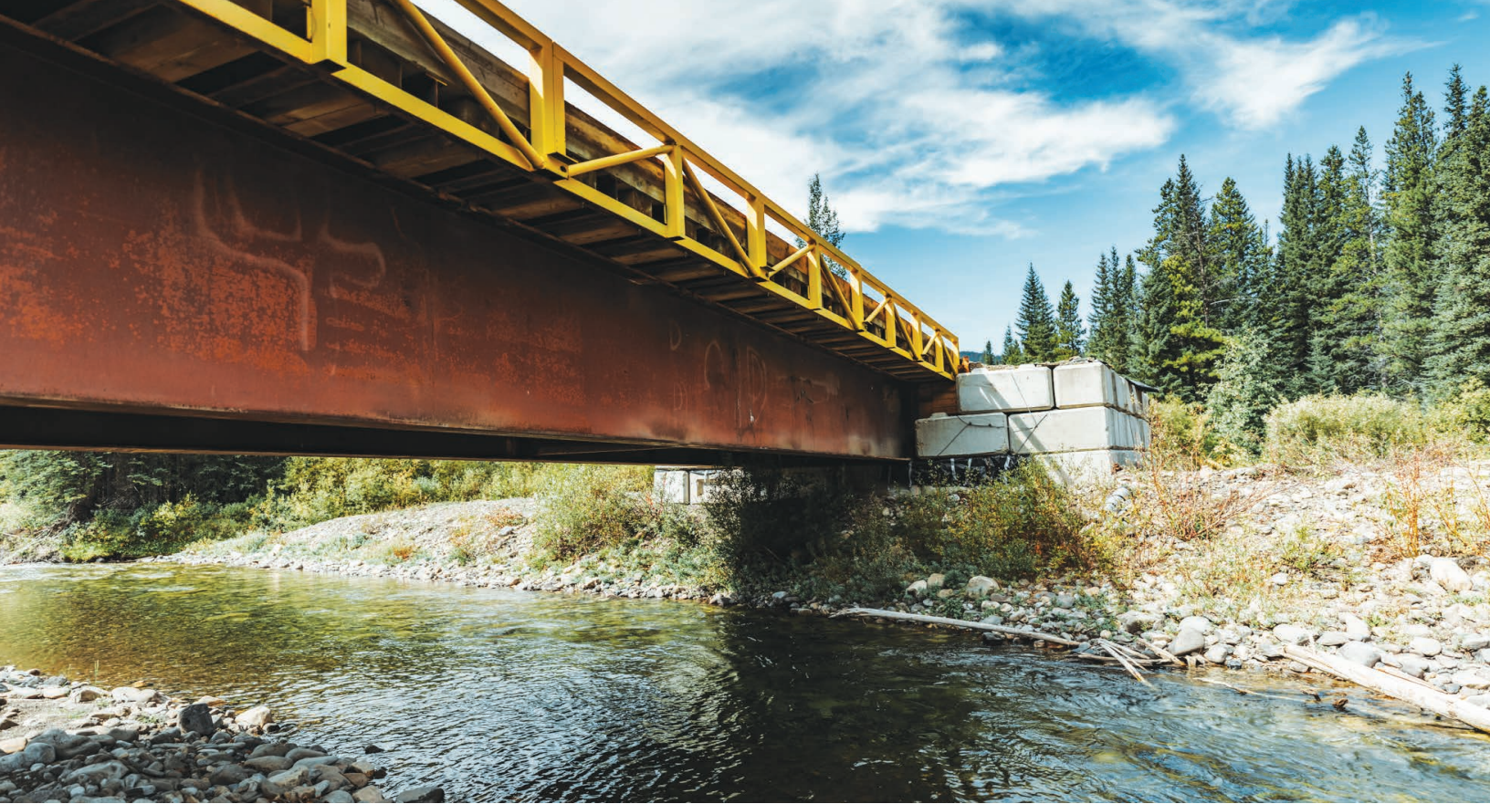
The bridge built over critical habitat for bull trout by Spray Lake Sawmills. Photo © A. Toner
