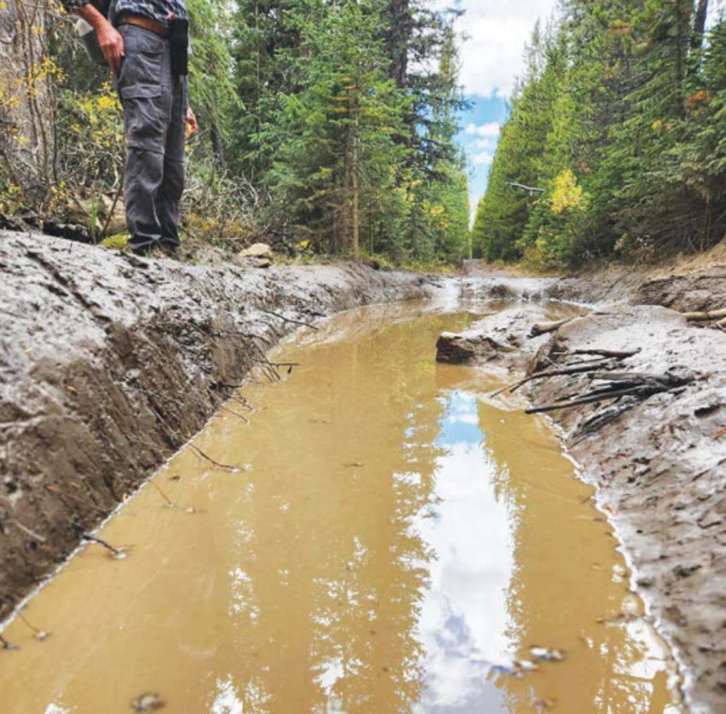
Deeply rutted, flooded OHV trails are the norm in the Hummingbird trail network. Photo © D. Earl
