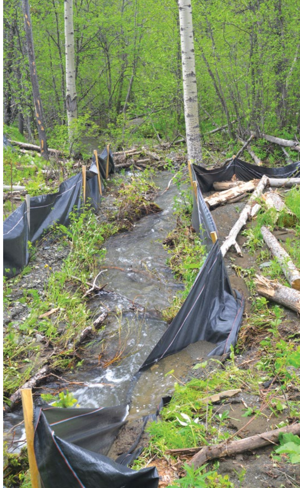
A collapsed sediment fence in Hidden Creek from 2013. Photo © L. Fitch
