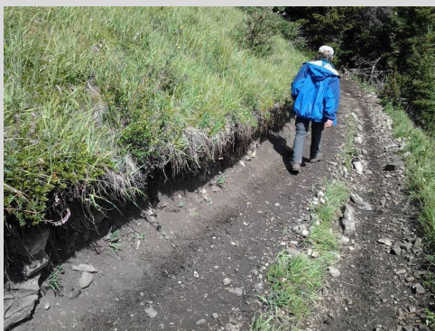
BTN damage site Taken 2015-07-16 Severity: 3 L: 80m, W: 1m, D: 100cm
