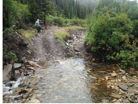
CAN water crossing Taken 2015-08-15 Severity: 5 L: 54m, W: 12m, D: 100cm
