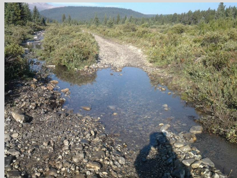
HUM water crossing Taken 2017-08-15 Severity: 1 L: 5m, W: 5m, D: 37cm
