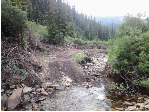
CAN water crossing Taken 2014-08-13 Severity: 5 L: 40m, W: 12m, D: 120cm
