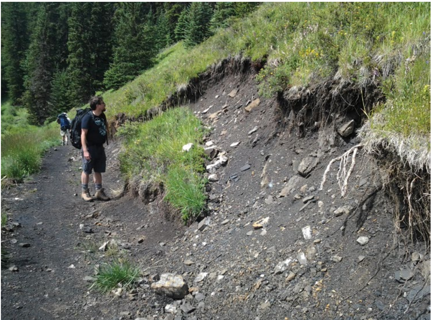
Slumping is a form of trail damage that occurs when a mass of land (i.e., dirt, clay, rocks, mud etc.) slides down a slope. This photo depicts an incident of slumping that was noticed during a trail survey in 2017. Photo © Alberta Wilderness Association.
