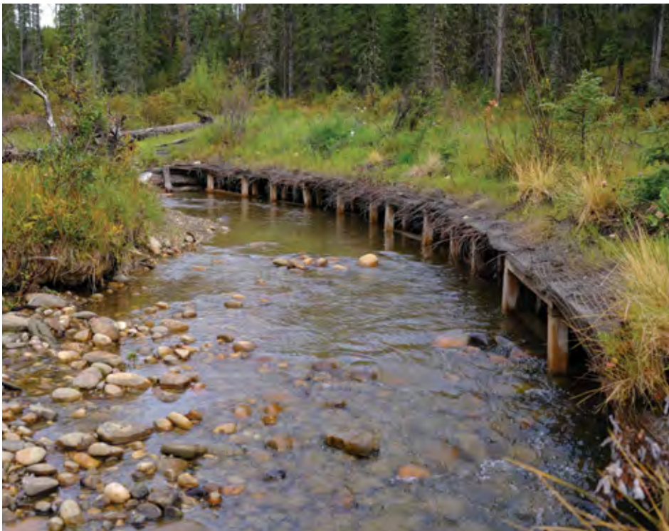
During AWA's site visit in September 2021, we were given a tour of the reconstruction efforts at various sections of Apetowun Creek that had been washed out by the coal mine spill, including the creation of artificial stream banks (pictured). Reconstruction efforts are now complete. Photo © P. Meintzer
