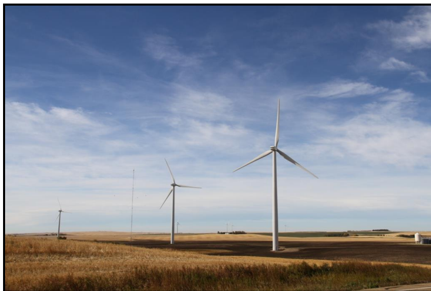
AWA continues to monitor new renewable energy projects and encourage development away from vulnerable locations, as well as supporting buffer zones for wind and solar farms.
