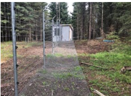
Perimeter fence, ground wire, and cub house. The ground wire is attached to the fence every 12 inches. It is now covered with soil so grass and other vegetation will grow there. PHOTO: © COCHRANE ECOLOGICAL INSTITUTE
