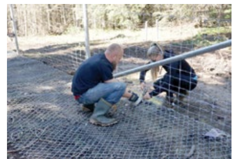
Volunteers attaching the ground wire to the perimeter fence. PHOTO: © COCHRANE ECOLOGICAL INSTITUTE
