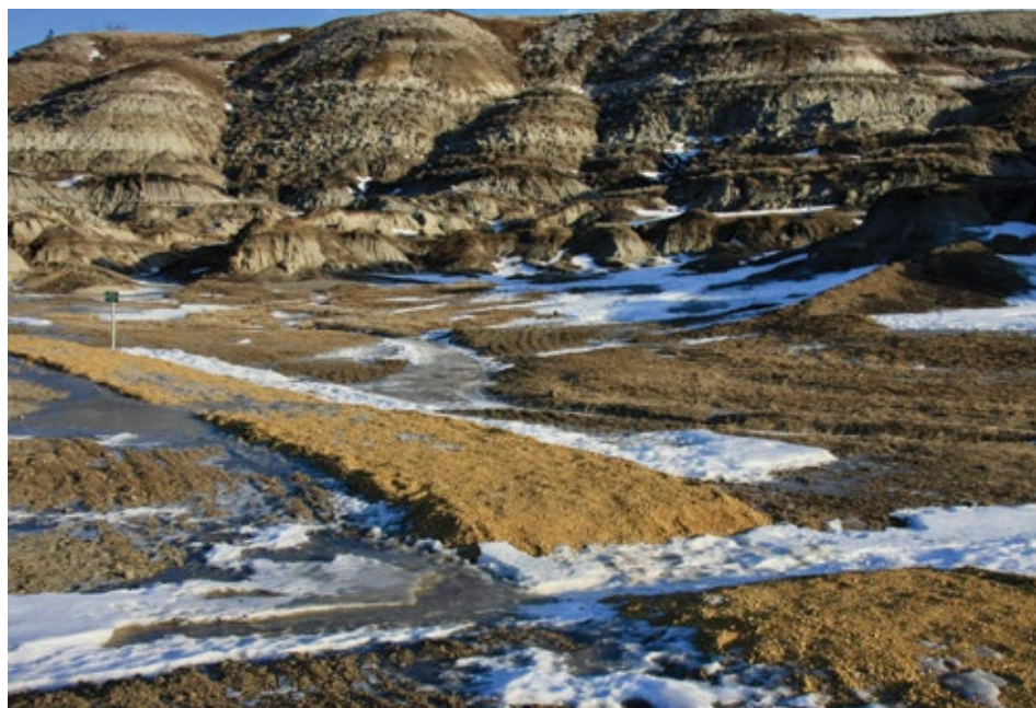
A closer look at the gravel road on the canyon floor. Note how raised the road is from the floor and how the road redirects surface water. PHOTO: © I. URQUHART
