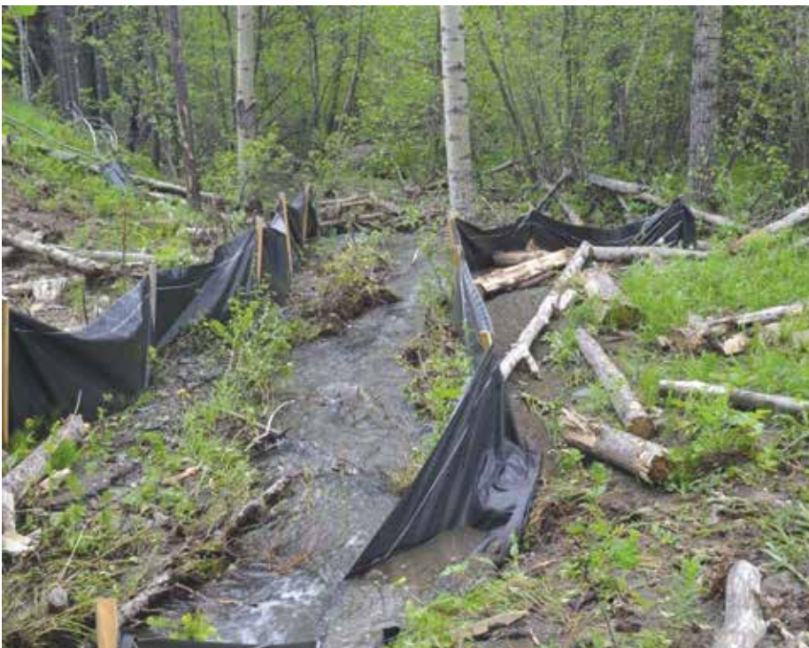
Sediment running off of cutblocks into Hidden Creek during the summer of 2013. The sediment retention barriers were clearly ineffective in preventing silt and mud from entering the creek. PHOTO: © L. FITCH.
