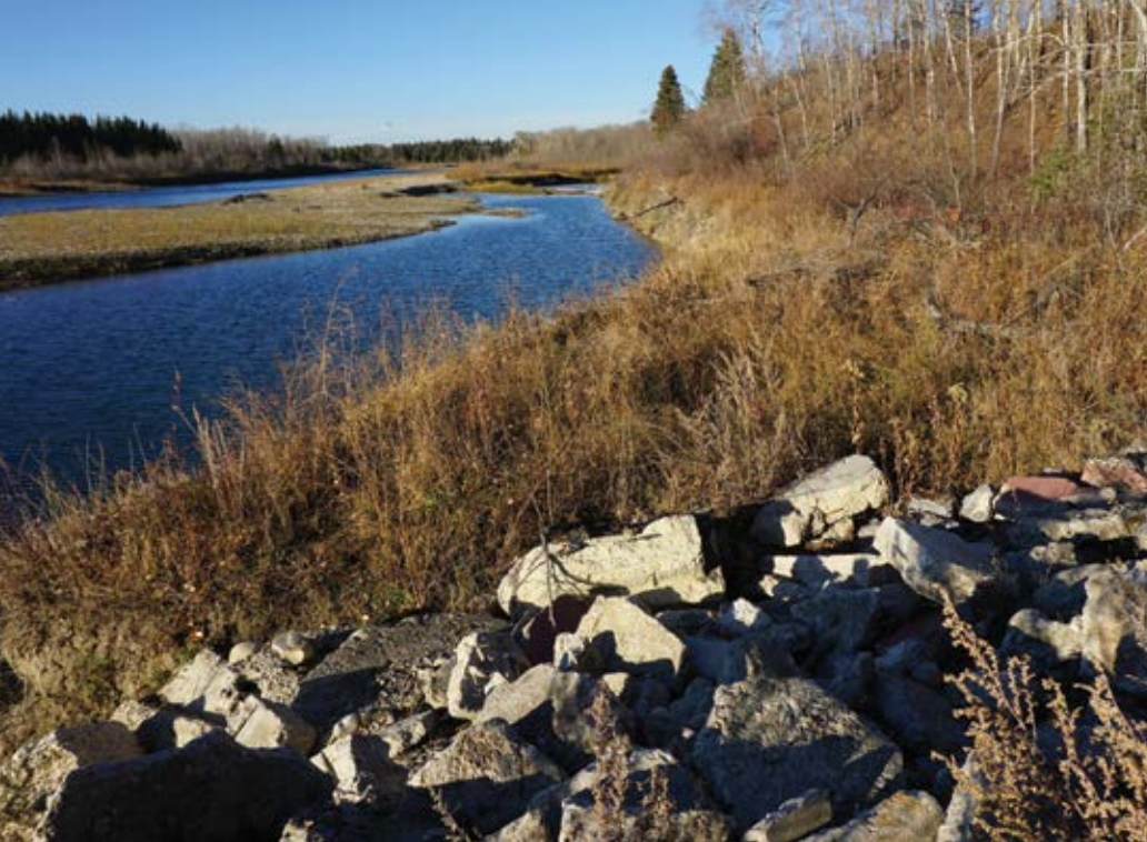
I took this photo of the interface between a gravel pit and a river in the fall of 2015. The riprap, rock used to armor streambanks, in the foreground of the photograph is the outer edge of the excavated pit. This pit has flooded numerous times, delivering high loads of sediment to the water. The river is very likely to overtake the pit again the next time it floods. PHOTO: © J. SKRAJNY
