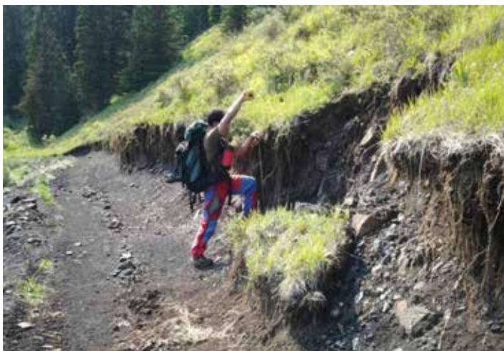
In 2015 volunteer Ken Lee measures collapsed sections of trail along Canary Creek, less than 10 months after the trail was constructed by the Government of Alberta. PHOTO: © S. NICHOLS
