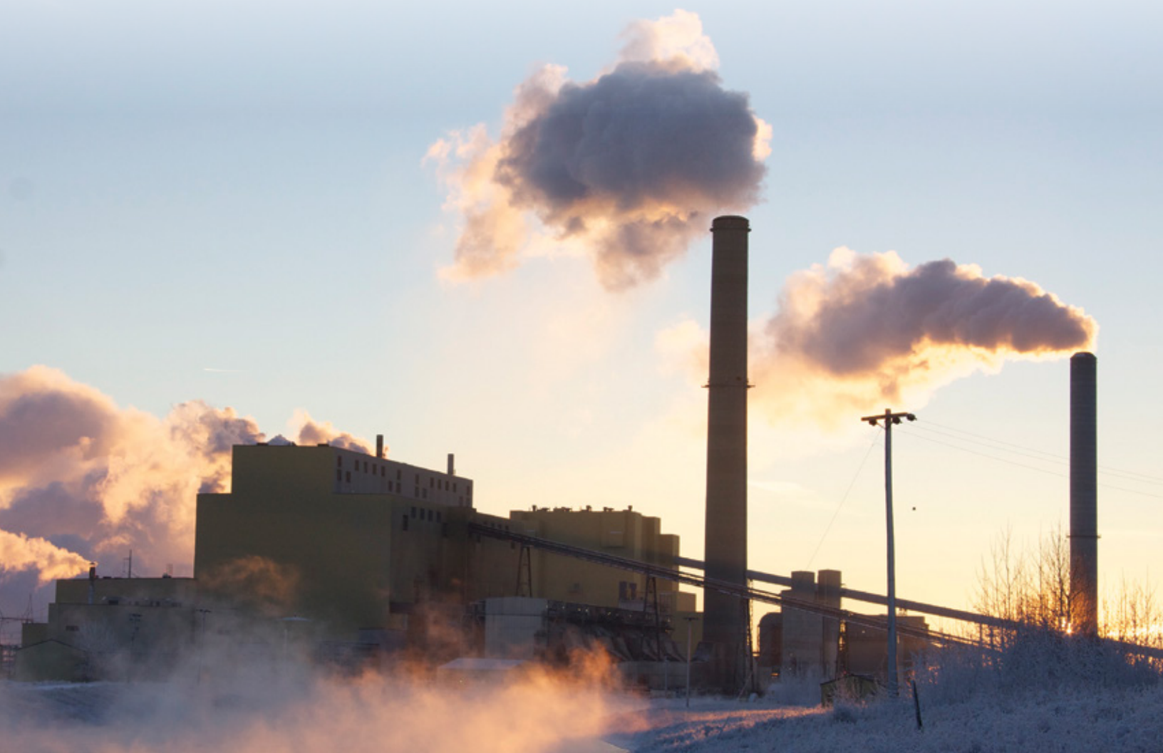
Keephills Generating Station PHOTO: © I. URQUHART
