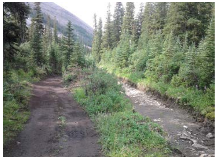
Here the trail, previously on the right of the photo, is now on the left. The trail on the left soon will likely look like the trail on the right. It too will exhibit root damage and dig-in. PHOTO: © S. NICHOLS
