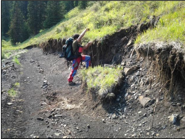
Slumping encountered on the Canary Creek trail less than 10 months after it was rebuilt under the BTFRP
