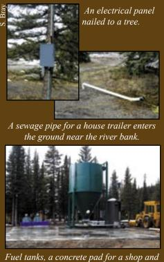
Fuel tanks, a concrete pad for a shop and a hopper that feeds fuel to an adjacent boiler at Panther River Adventures
