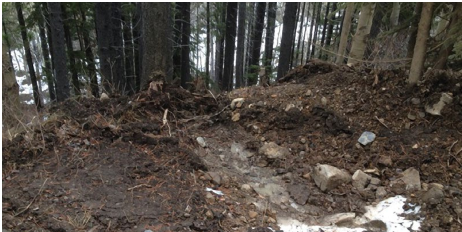
A breach in the Star Creek haul road's meager berm allows muddy water to flow down into Girardi Creek, about 20 metres distant. PHOTO: © D. MCINTYRE
