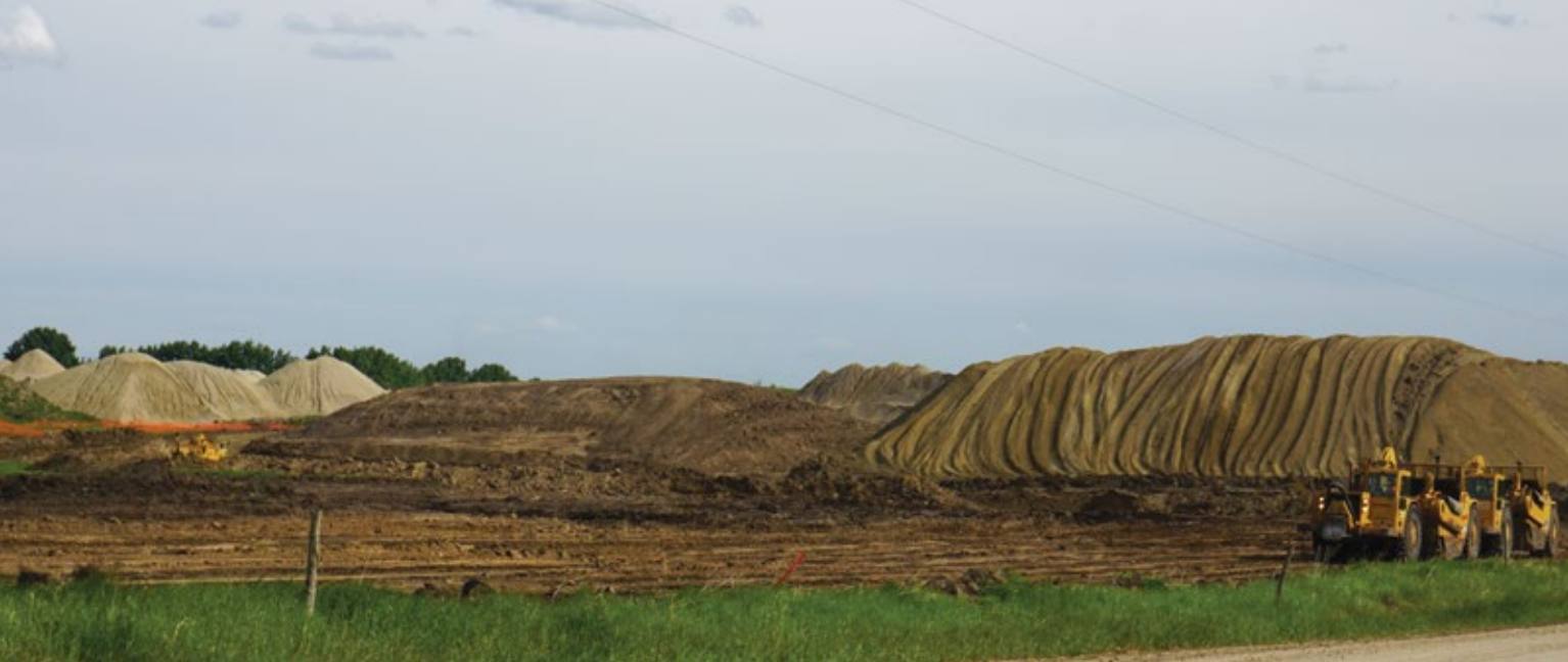
This gravel extraction site on higher ground will likely interfere less with groundwater than the ones further down in the floodplain. The piles of sand and clay left after washing still present reclamation challenges, such as how water drainage on the reclaimed topography will affect natural water bodies. PHOTO: © C. CAMPBELL
