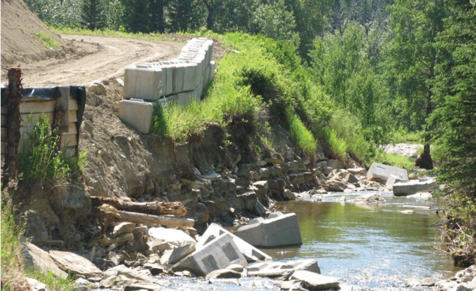
Poor logging practices, seen here in the absence of any vegetation buffer along a road built by Spray Lakes Sawmills in the Porcupine Hills, leads to erosion into the adjoining stream. PHOTO: © G. RIDDELL
