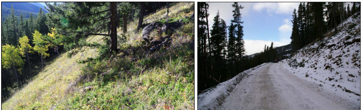
Figure 3: Access road cutting across steep slope down to Hidden Creek: before and after. What kind of erosion can be expected to occur here? How will this be reclaimed to its pre-development state? What does this mean for sedimentation of the creek?
