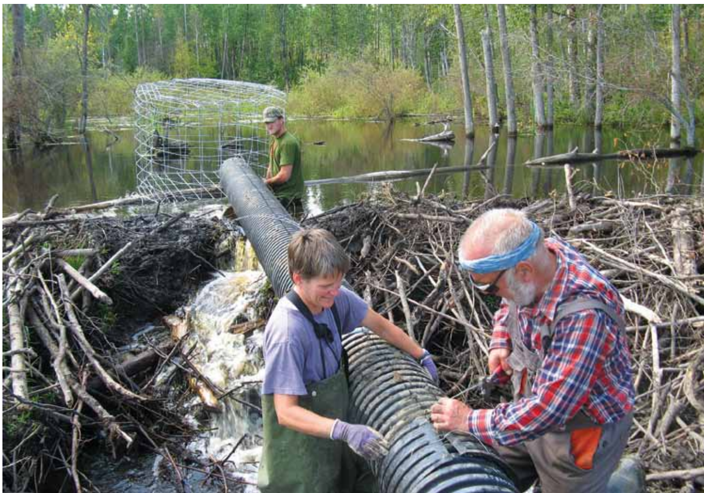
Installing a pond leveler to maintain water levels and prevent flooding of trails in the Cooking Lake/Blackfoot Provincial Recreation Area.
