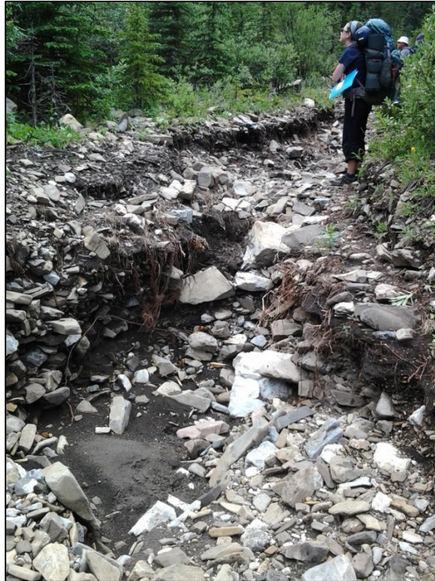
Figure 4. A section along CAN trail showing a damaged site of approximately 1.75 m in depth.
