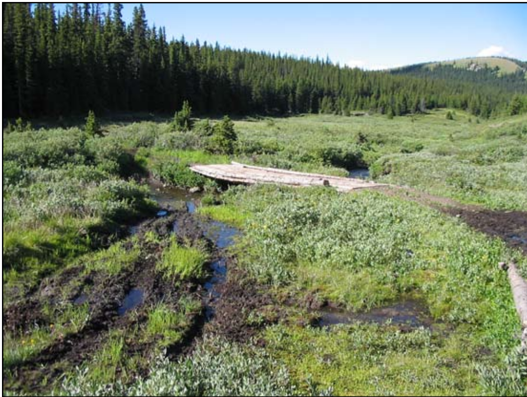
Figure 7. A water crossing on BTN. The bridge was placed on the main trail, but users continue to drive OHVs through the creek on the left side of the photo.
