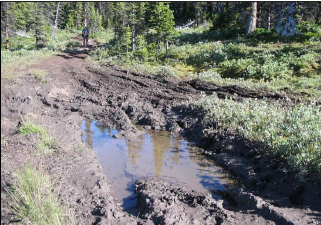
Figure 9. Trail degradation due to a combination of poor water drainage and excessive motorized traffic. Pooling water in one section of the trail leads to trail braiding and exacerbates vegetation loss and soil erosion.
