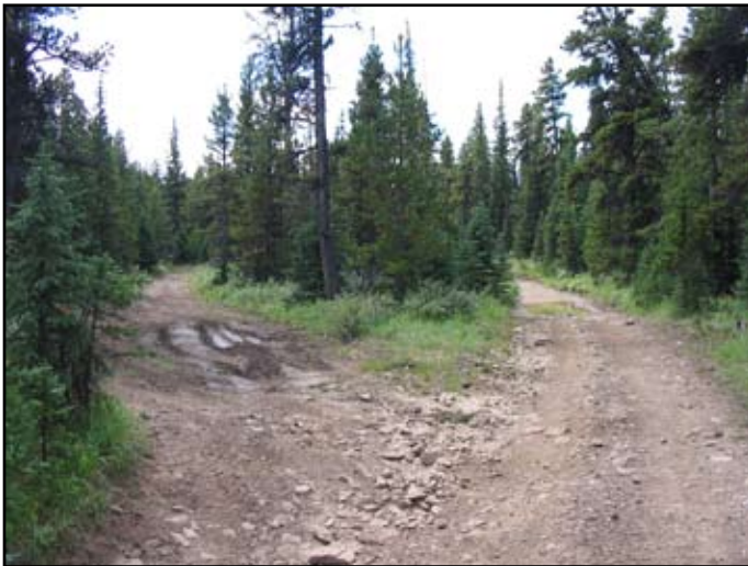
4) Trail braiding along the ONC trail. Note the puddling on the left branch.
