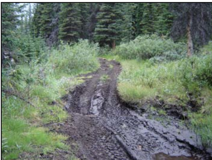
5) A section of damaged trail along HUM. Poor trail construction is leading to water pooling and rutting along this OHV track.
