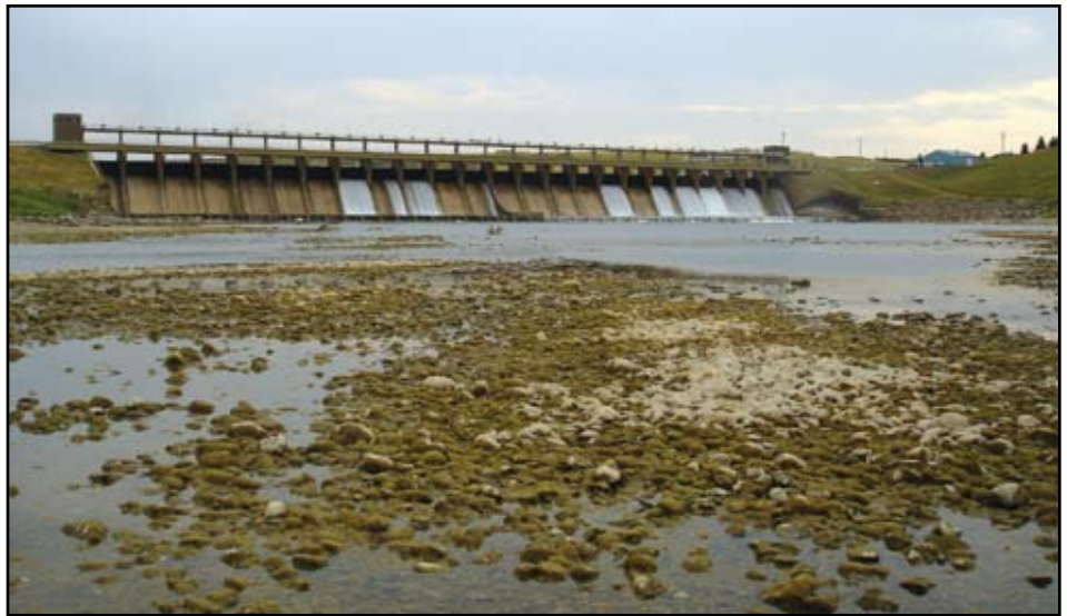
Bassano Dam is where the Eastern Irrigation District withdraws water from the Bow River. These withdrawals cause extremely low flows in late summer. On this day, August 9, 2006, the flow below Bassano Dam was 9 m 3 /sec; the flow in Calgary (above all irrigation diversions) on that day was 82 m 3 /sec. PHOTO: WATER MATTERS
