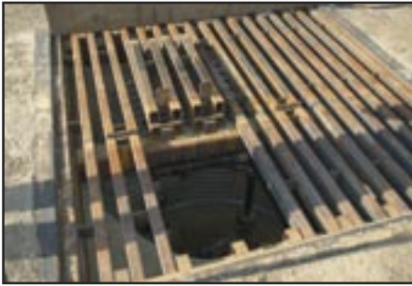
An example of a sunken well head in the Suffield block. The wellhead is covered with sturdy metal bars and plywood that can withstand the weight of passing tanks.
