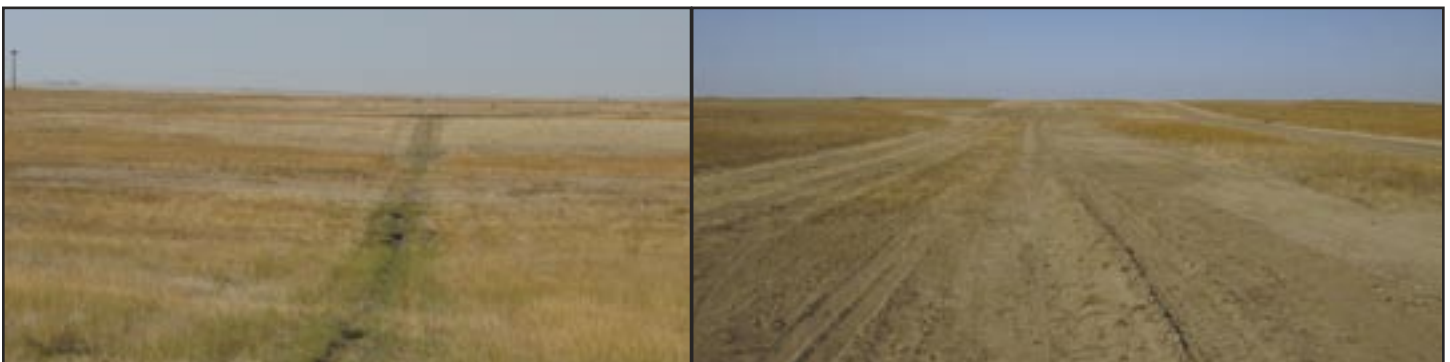
These photos, both taken in September 2006 on a field trip with EnCana, show the difference in disturbance from ploughing in (left) and trenching in (right) a pipeline. Although both can recover naturally, this trenched-in pipeline must be reseeded because of the proximity of crested wheatgrass, an invasive species. EnCana's infill project in the Suffield National Wildlife Area plans 180 km of 5-inch plastic pipeline that can be ploughed in and 40 km of 16- to 20-inch steel pipe that must be trenched in.
