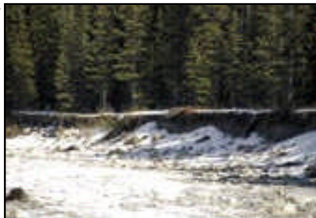
The southern bank of the Panther River adjacent to the proposed expansion shows erosion from the river.
