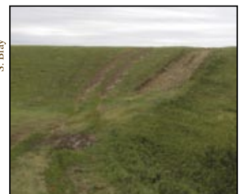
Erosion from vehicles on a hillside in the Rumsey Natural Area
