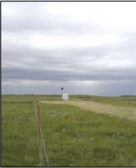
Trident's first CBM wellsite in the Rumsey Natural Area showing the pipeline path seeded with annual rye
