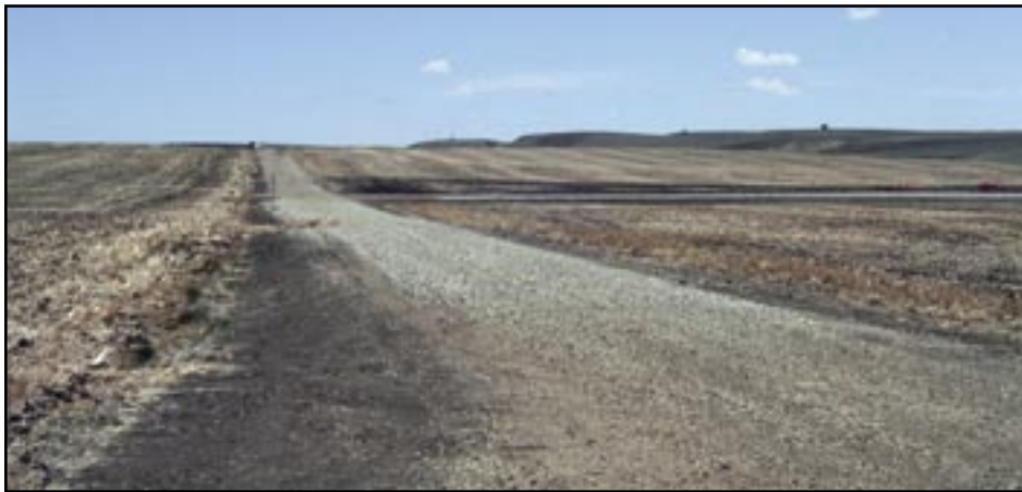
A 1100m long lease road to a CBM well.
