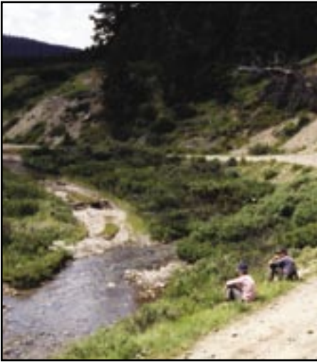
An OHV trail bypasses the main route and goes through a stream. The stream bed has widened due to erosion.
