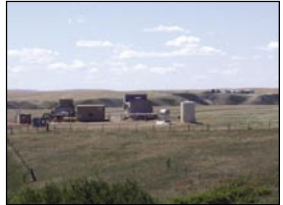
Compressors two miles northeast of Rosebud. There are two additional compressors less than one mile northwest of Rosebud.
