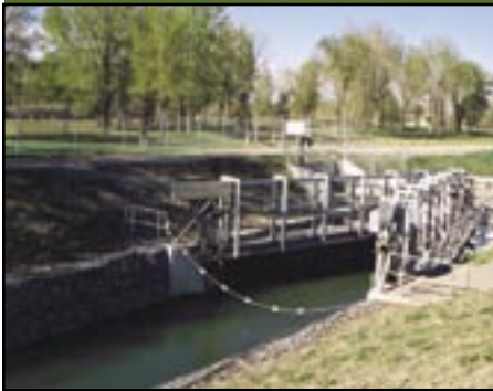
Both the Pine Coulee and Little Bow projects included fish screens, metal structures intended to prevent fish passage into the diversion canals. This photograph shows the fish screen in the Little Bow Canal in the Town of High River that traps large and even fairly small fish, which are then flushed back into the Highwood River
