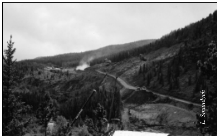
Cardinal River Operations haul road and public road from the Luscar Mine site up the McLeod valley towards the old mine village of Mountain Park in the middle of its Cheviot Mine permit area. Access from Cadomin to Whitehorse Creek campground and the Mountain Park area has been restricted, except on long weekends when CRO has been providing escorted access. Due to weather and other delays, the re-opening of the public road may not be until about mid-September.
