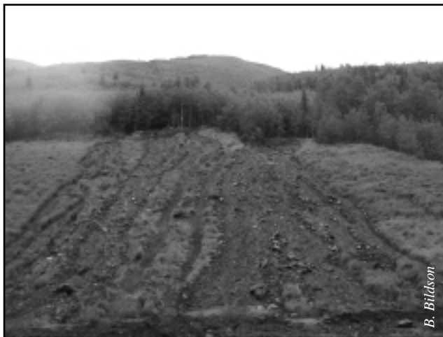
An example of the slope instability at an abandoned Smoky River Coal Site at Caw Ridge
