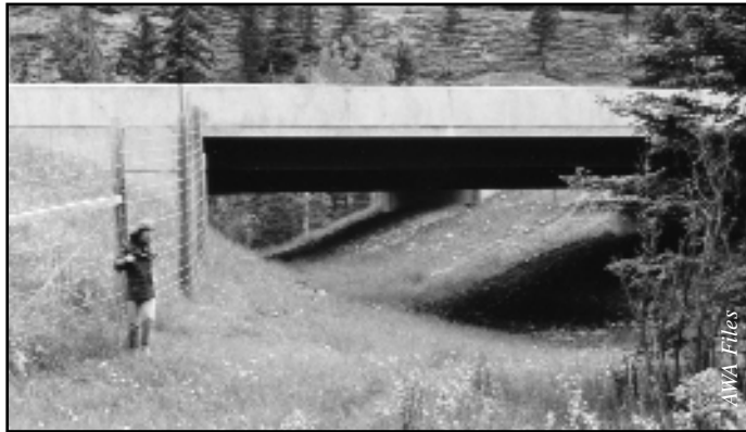
Highway underpass for wildlife along TransCanada Highway in Banff National Park
