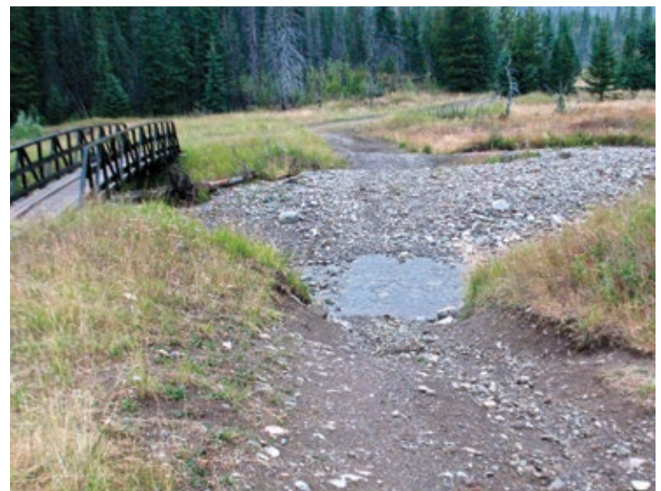
Freshly-used OHV ford over Lynx Creek, within designated westslope cutthroat trout critical habitat, immediately beside a brand new OHV bridge. PHOTO: © D. MAYHOOD
