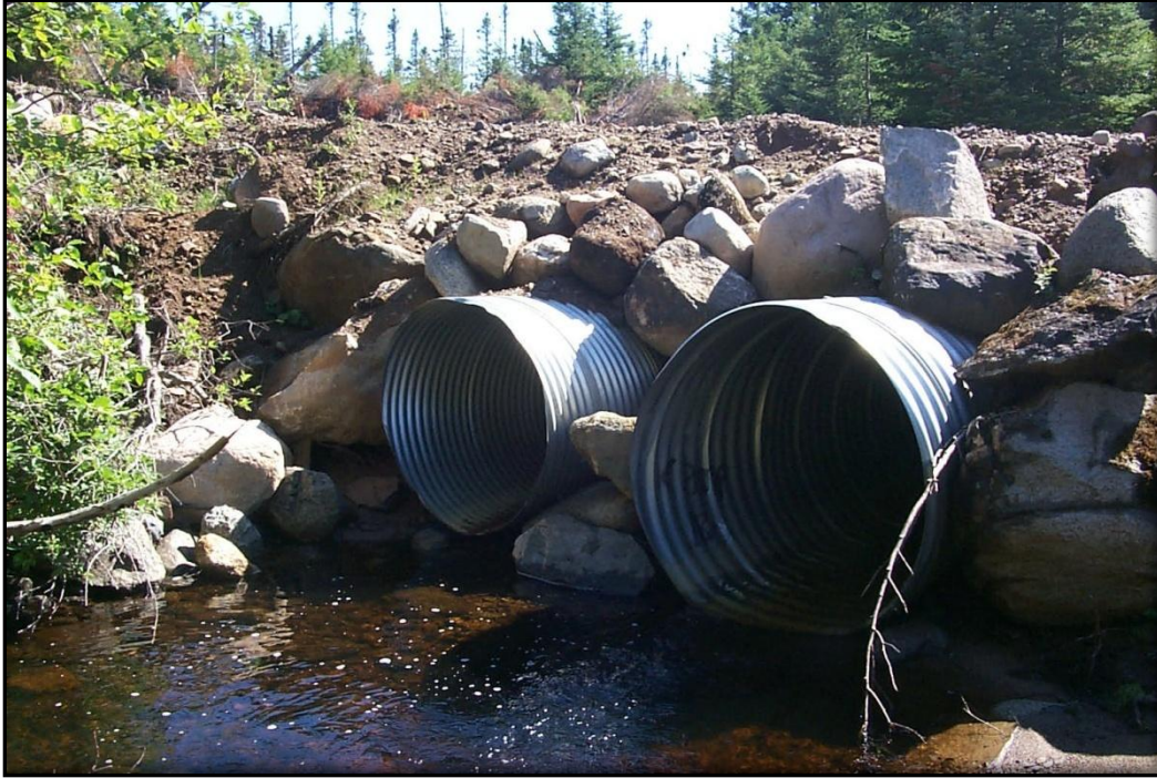
Figure 11. An example of a hung culvert that interferes with fish movement. Photo courtesy of Dr. Michael Sullivan (Government of Alberta).
