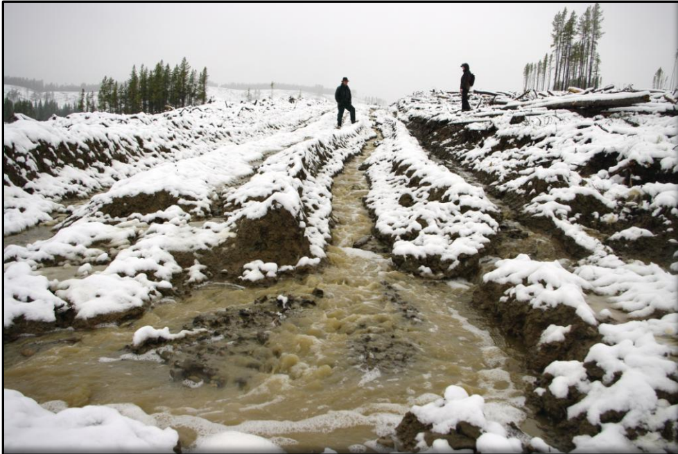
Figure 18. Sediment erosion from inblock road, Meadow Creek area cutblock, Ghost River study area, 27 May 2011.
