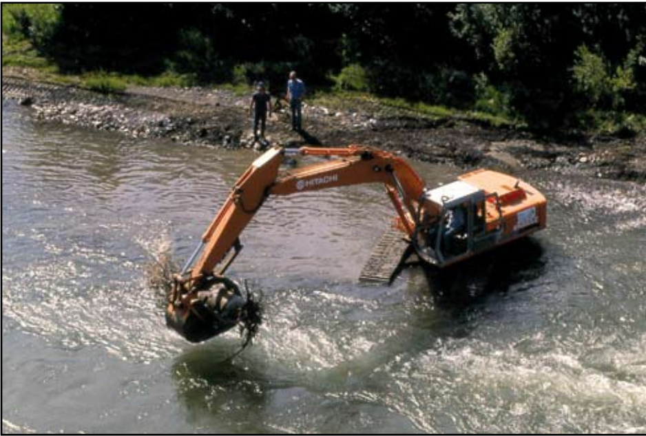
To mitigate the effects of the Oldman Dam, an attempt was made to create deep-water trout habitat in the Crowsnest River. Six years later, only a third of the new habitat remained, and this remnant may not meet the criteria for good-quality deep-water habitat. PHOTO: L. FITCH
