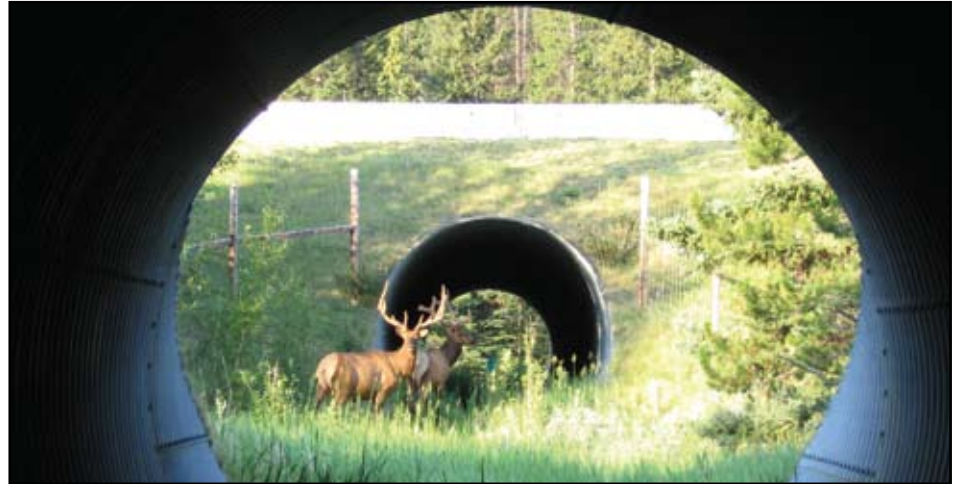
Two elk contemplate using one of the underpasses in Banff National Park to cross the Trans-Canada Highway. PHOTO: A. FORD/WTI
