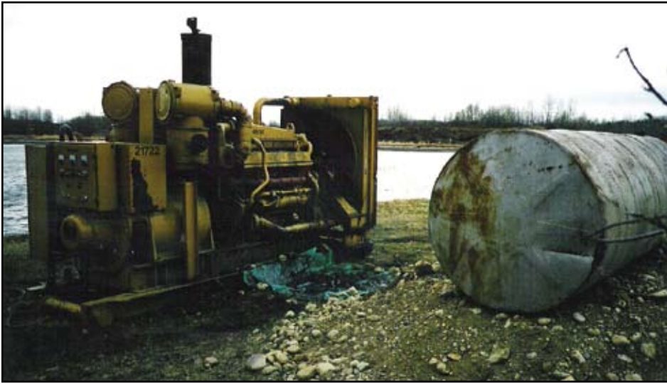
An unlawful operation identified by ORVCA in May 2001, which has since been rectified. As part of a gravel mining operation, a generator engine for pumping water stands at the edge of an exposed aquifer reservoir. The blue canvas catches raw petroleum products leaking from the engine. Neither the engine nor the nearby 4,000-litre diesel fuel tank had any containment structures in case of a fuel spill.
